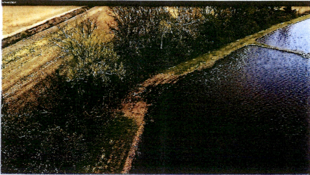
Photo 5. Helena WWTP Cell 3 South-west corner aerial view
